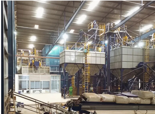
ROOF ELEVATION, MACHINERY FOUNDATIONS & PARTITIONING AT ETG
