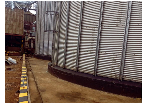
UGACOF COFFEE PROCESSING PLANT ENHANCEMENT, BWEYOG...
