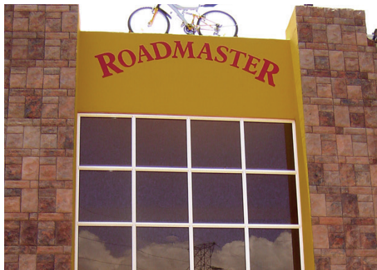
CONSTRUCTION OF ROAD MASTER CYCLES PAVILION, LUGOGO
