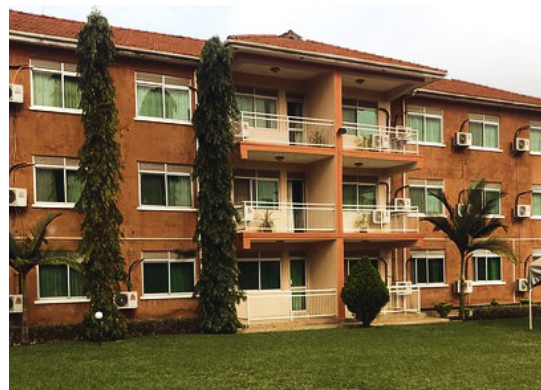
CONSTRUCTION OF GULU CHURCHILL COURTS HOTEL
