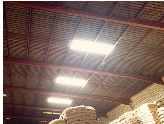
DIVERSE CIVIL WORKS FOR OLAM, NAMANVE
