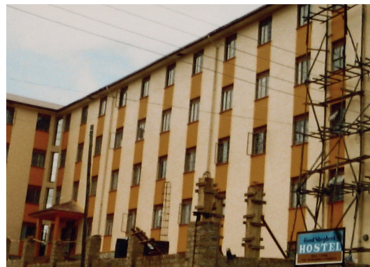
CONSTRUCTION OF GOOD SHEPHERD HOSTEL, BANDA
